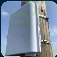
Fiber optic joint closure fixation
